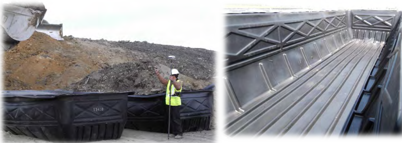
Figure 10. Polyethylene Sealed container for Landfilling BSE-Infected Carcasses (Photos courtesy of USDA APHIS Veterinary Services, Blue Incident Management Team, 2012).
